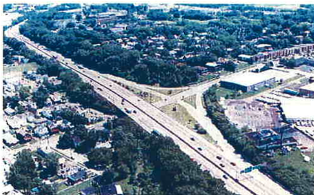
Towne Street Interchange (photo by Larry Stulz)
