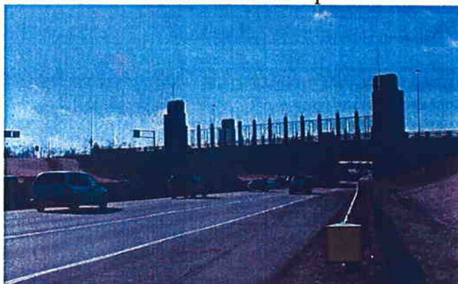
Recently completed Paddock Road bridge
